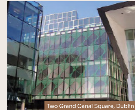
Two Grand Canal Square, Dublin 2
